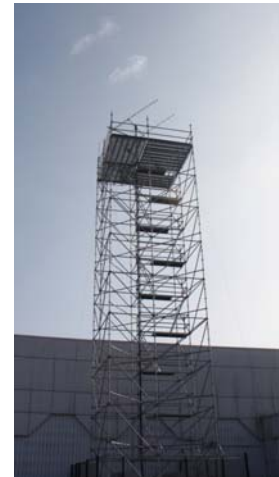
Antenna tower in Redu.
